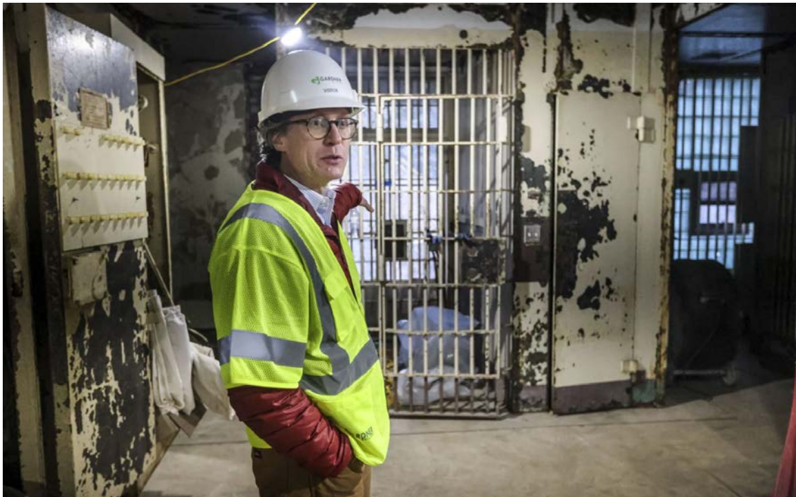
Leijona developer Jon Commers describes an area of the fourth-floor jail block in 2021, at the former St. Louis County Jail in Duluth. Clint Austin / 2021 File / Duluth News Tribune
