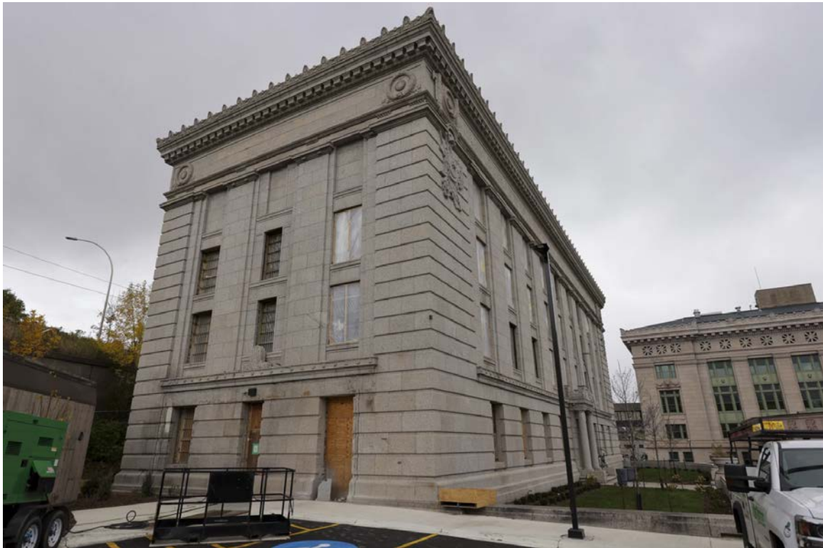
The exterior of the Leijona apartment complex under construction in the historic St. Louis County Jail building on Oct. 13 in Duluth.
